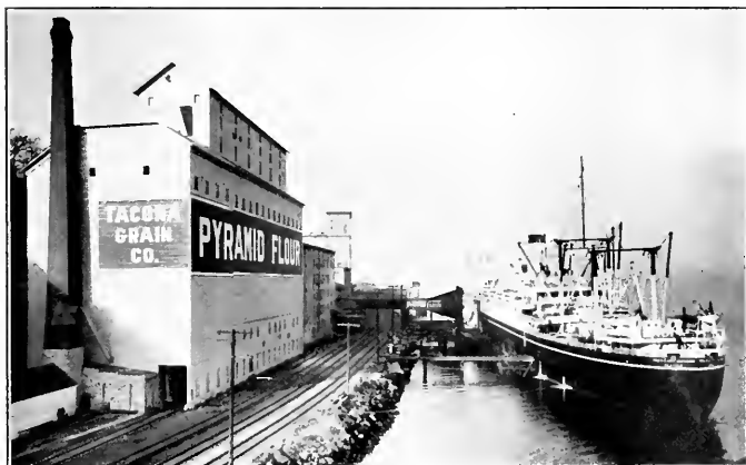
Picture shows the Dollar Liner President Jackson alongside the Tacoma grain pier at Tacoma, Washington, in December. She is taking on the first cargo of wheat and flour shipped from that terminal after completion of its alterations and enlargements made during 1930. The main line tracks are shown running on fill where the old dock formerly stood. Forty-five feet of water at the ship's position.
